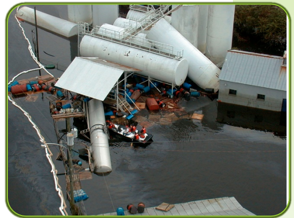
In 1999, flooding from Hurricane Floyd toppled storage tanks and carried away oil drums, resulting in floodwater contamination in Franklin, Virginia. Credit: Liz Roll/FEMA News Photo.
