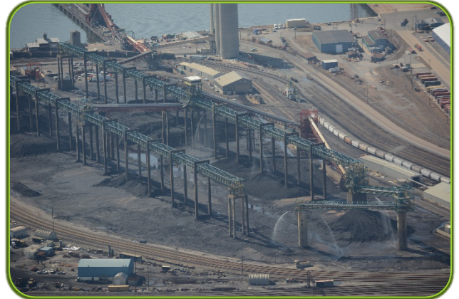
Dominion Coal Terminal in Newport News, Virginia. Credit: James River Association.
